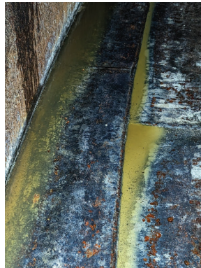
Liquid still present in the weld seams.
