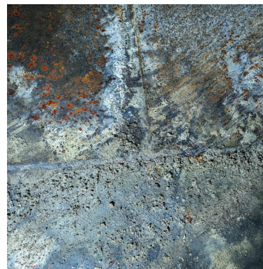
Product residue still present on top of floor plates
