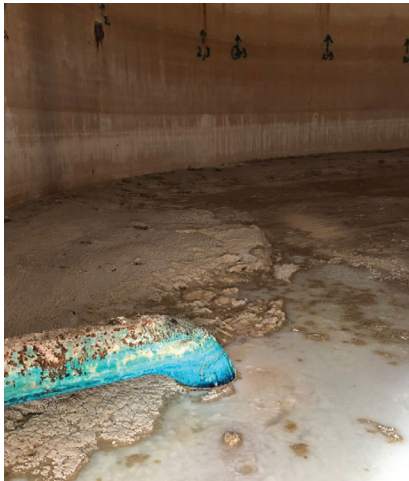
An example of a tank that is generally not cleaned properly.
