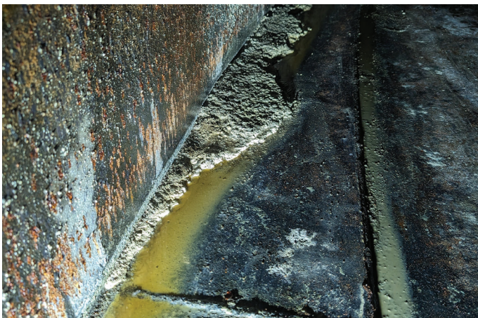
Excessive scale build up along the inside chime well. This is considered a critical zone of the tank due to it being the highest pressure area inside the tank.
